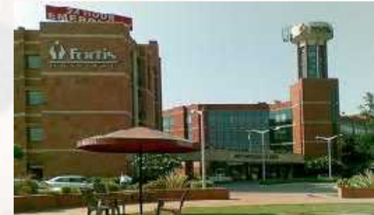
Fortis Hospital, Mohali
